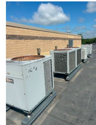
Condensing units serving the G-Wing district and activities offices, and band and choir. Condensing units age 34 years. Life expectancy 15-20 years.
