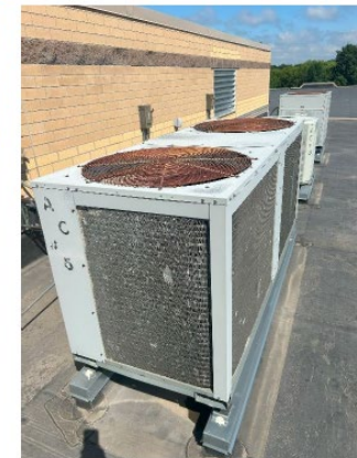
Condensing units serving the G-Wing district and activities offices, and band and choir. Condensing units age 34 years. Life expectancy 15-20 years.
